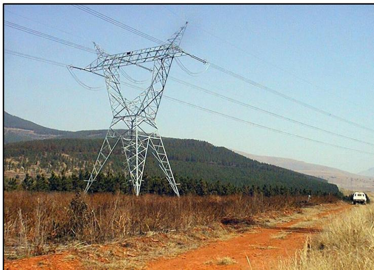
**Figure 3: Self-Supporting Strain Tower**
